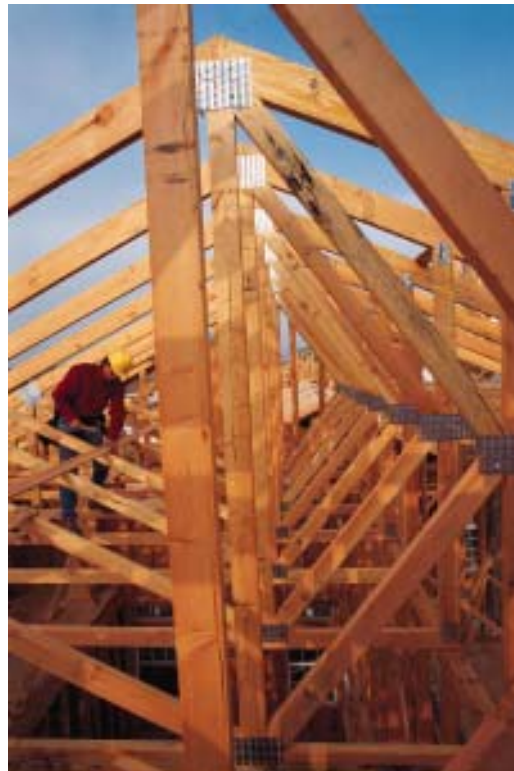
Trusses manufactured in the NWT
