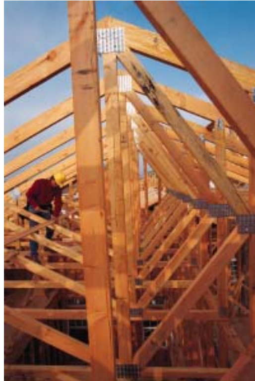
Trusses manufactured in the NWT
