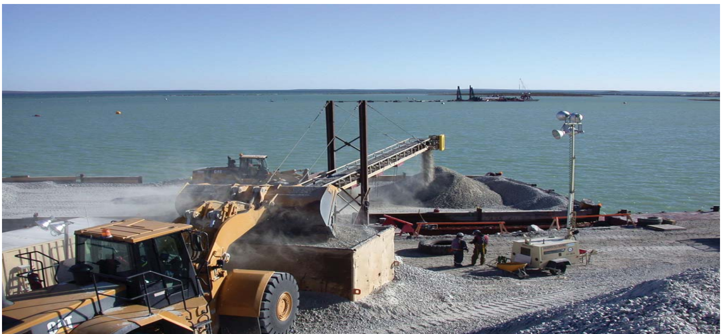
Building of the Dyke at the Diavik™ Diamond Mine
