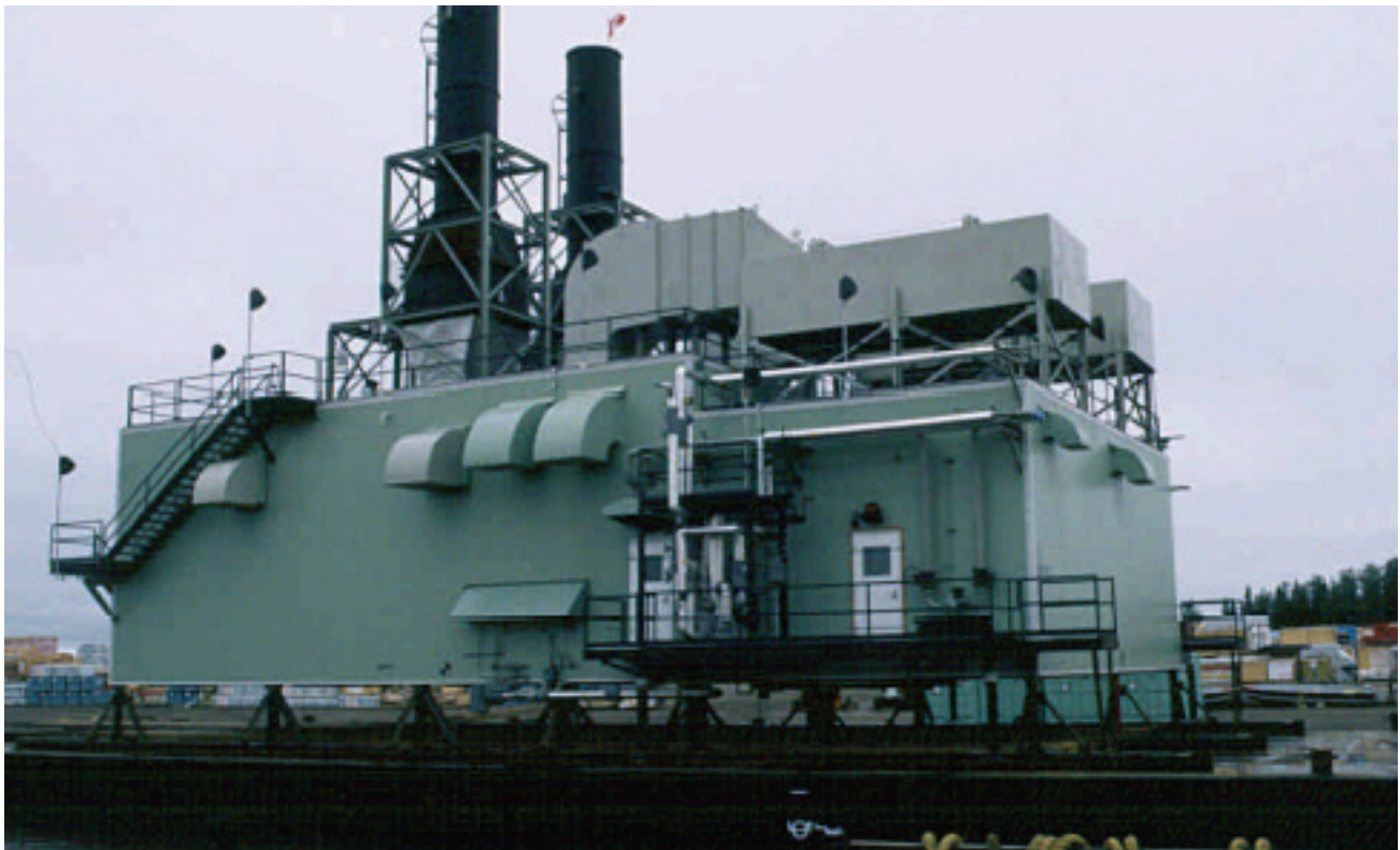
Source: Transport Canada; Oil field module destined for Alaska via the Mackenzie River Barge and Rail system
