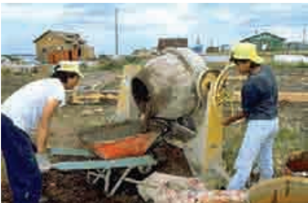
Source: ITI - GNWT, Batching Concrete in Behchokò
