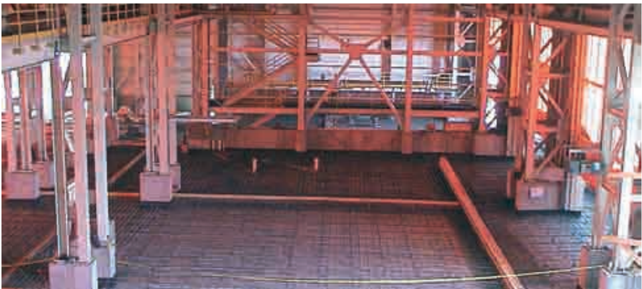
Source: Diavik, Shop Construction
